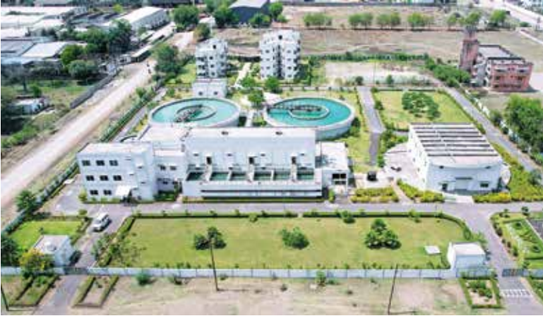
▲ Dewas industrial area water supply project, Madhya Pradesh.
