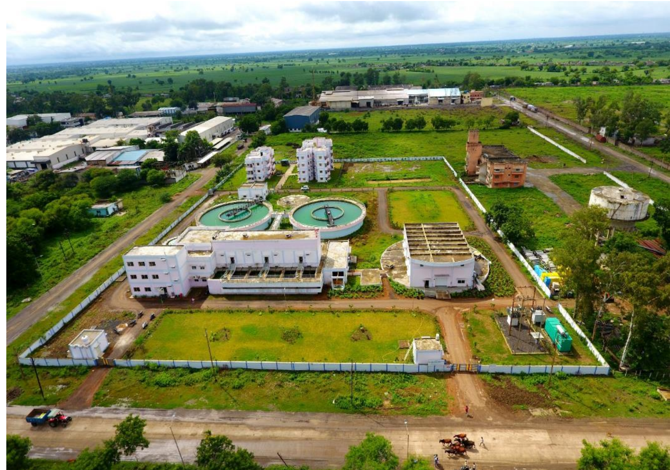
Industrial Water Treatment Plant, Dewas, Madhya Pradesh
