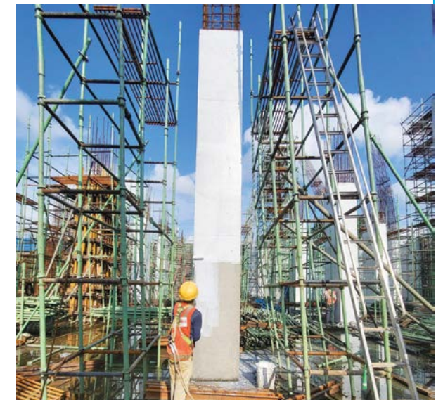
» Acrylic-based curing compound application
