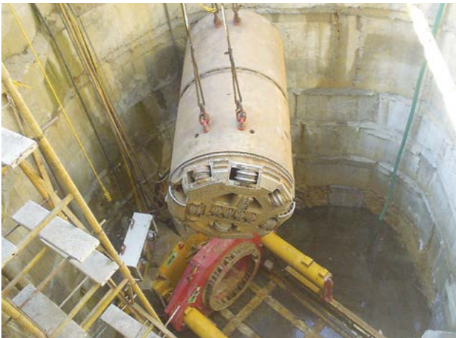
» Microtunnelling Project, Mumbai
