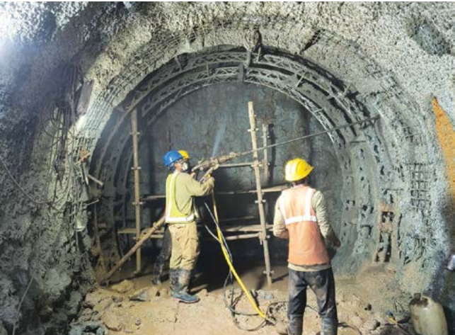
» Priority Sewer Tunnel Phase-I (PST-1) Project, Mumbai
