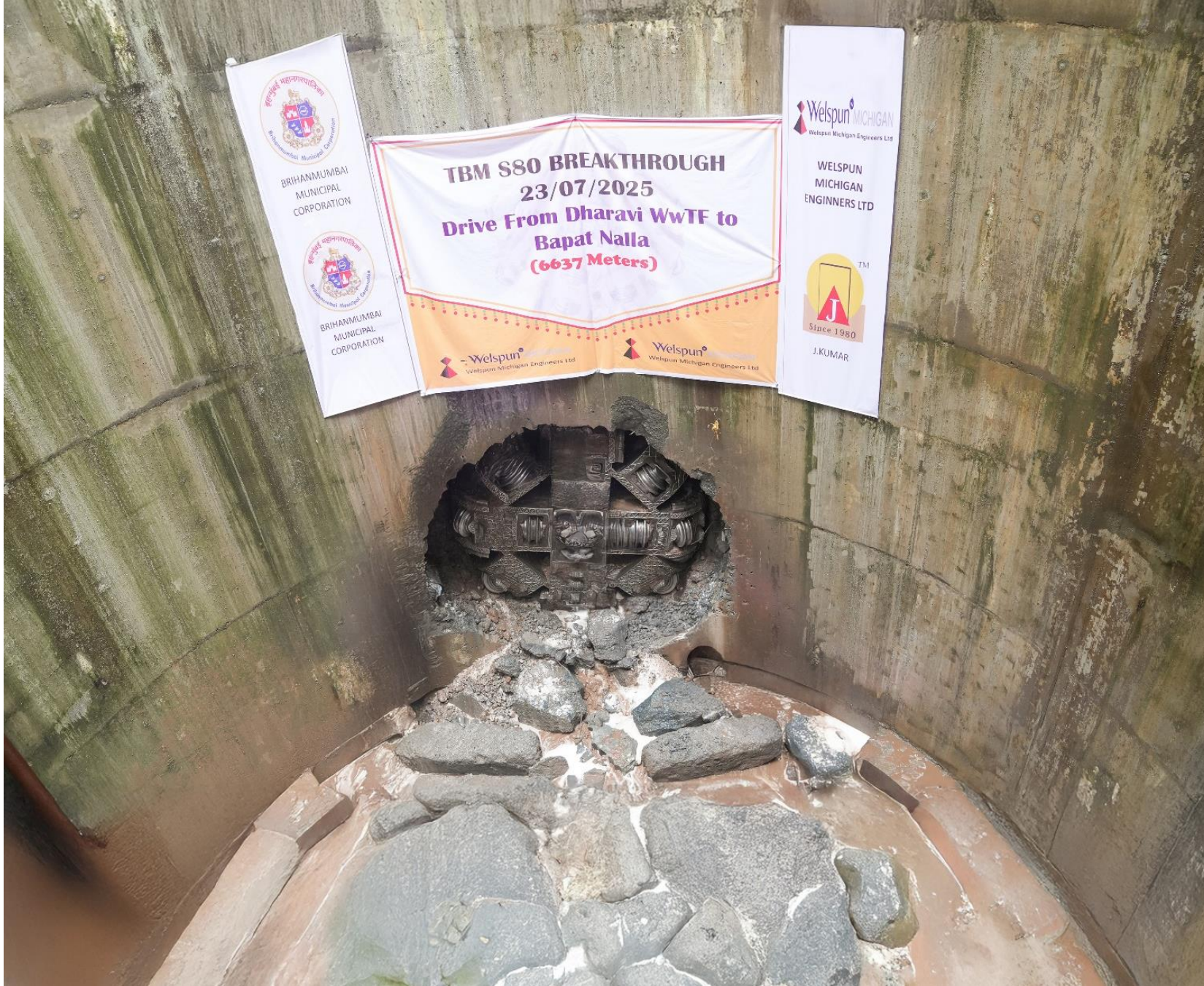
Mithi River Tunnel Breakthrough
