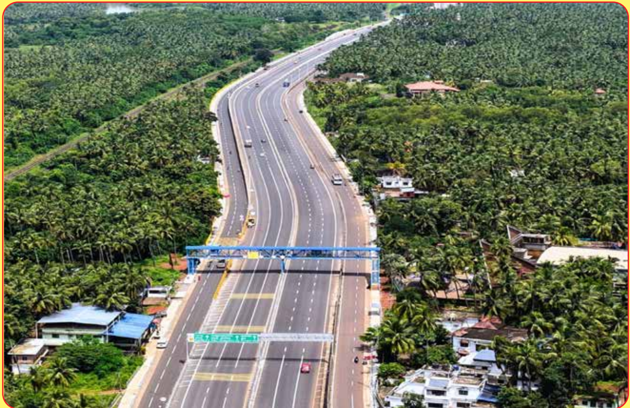
A View of National Highway-66 (Thalappady–Chengala Section) in the State of Kerala
