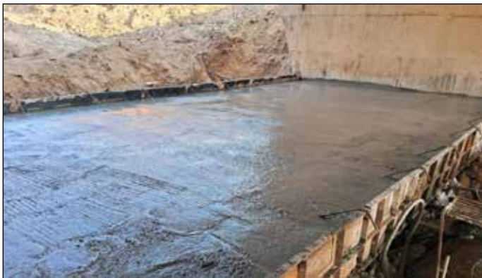
Fig.29 Pile Cap Casted to Complete Integration of Pile with the Box
