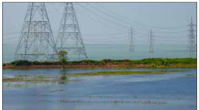
Fig. 4 Water-logged Area of RUB1-RUB2-ROB stretch (Image taken towards RUB1 from top of Railway Embankment at RUB2 location)
