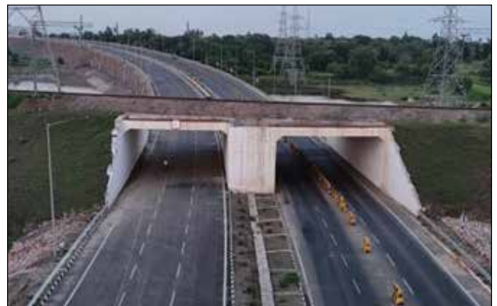
Fig. 31 Showing Underpass after Finishing
