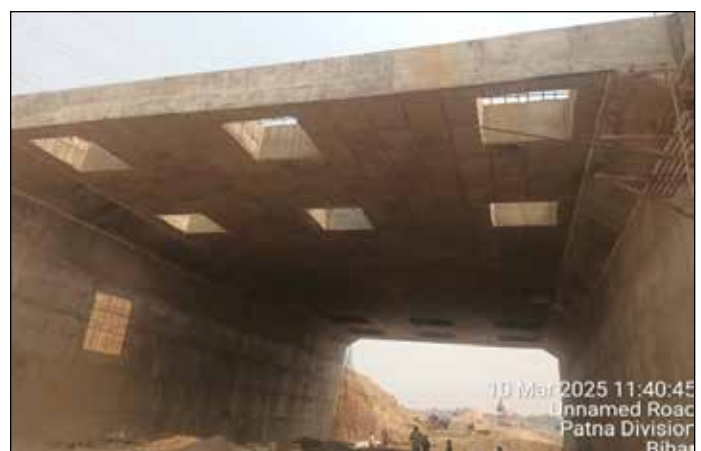
Fig.27 Pockets Left in Top Slab for Piling
